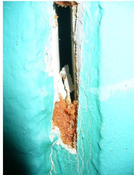
Dehnfuge asbestfrei, PCB-frei
